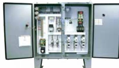
monitor, the control box can be remote mounted up to 1,000-feet away or mounted at the dryer. The touch screen communicates with the dryer power box via an ethernet communication link.
